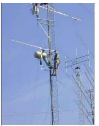
Above: Adjusting the 24 gHz dish at K1WHS-with 1296 loop to peak the pointing.
